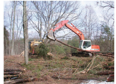
Tree trunks were ground with a level grinder and removed from the site
